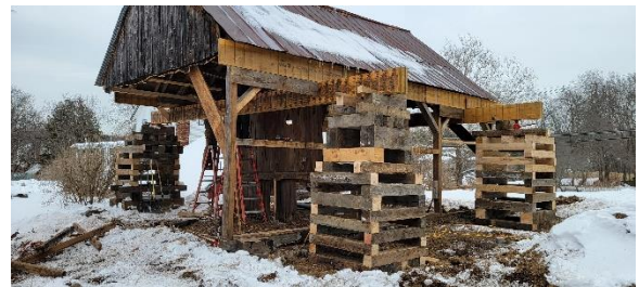
The old shed jacked up on temporary supports during restoration.
