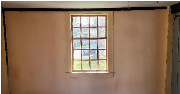
Association Room - Newly plastered walls and ceiling with new trim on windows and corner posts.
