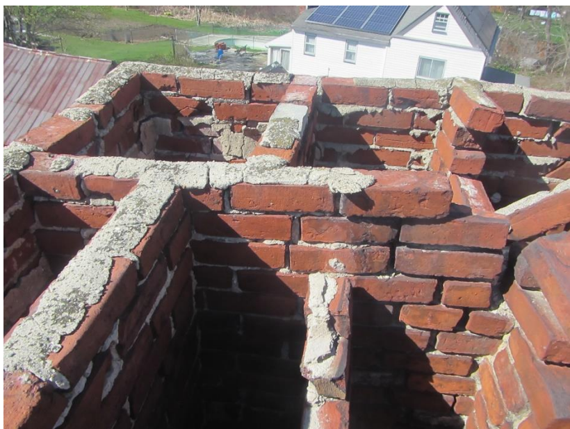
Chimney prior to repair.
